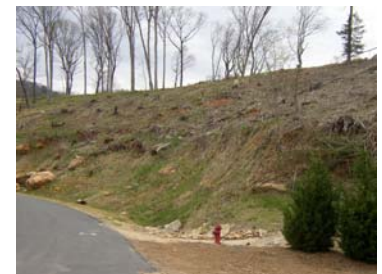
Development, road construction, and removal of vegetation adversely affect erosion. Exposed soils allow stormwater to gain velocity during precipitation events; the stormwater gathers sediment and pollutants and carries them into streams, creeks, and lakes.
