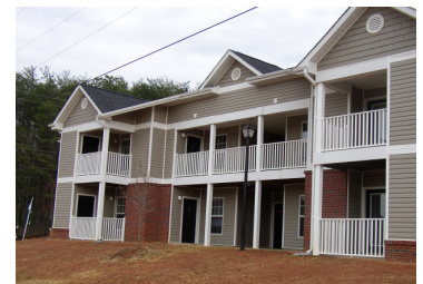
A multi-family development in Lake Lure: apartments located near the Ingles grocery store.
