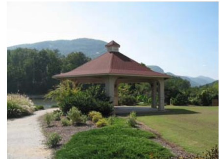
The Public Works department maintains Morse Park's grounds and structures.
