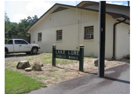
Location of maintenance facility could be utilized better by commercial development.
