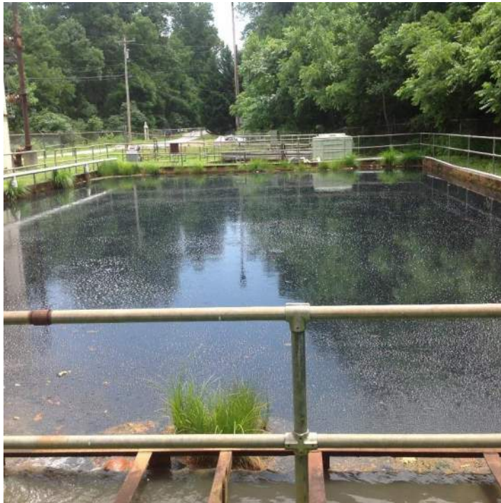
Sedimentation Basin with heavy solids deposition due to P/C Process and non-functioning digester
